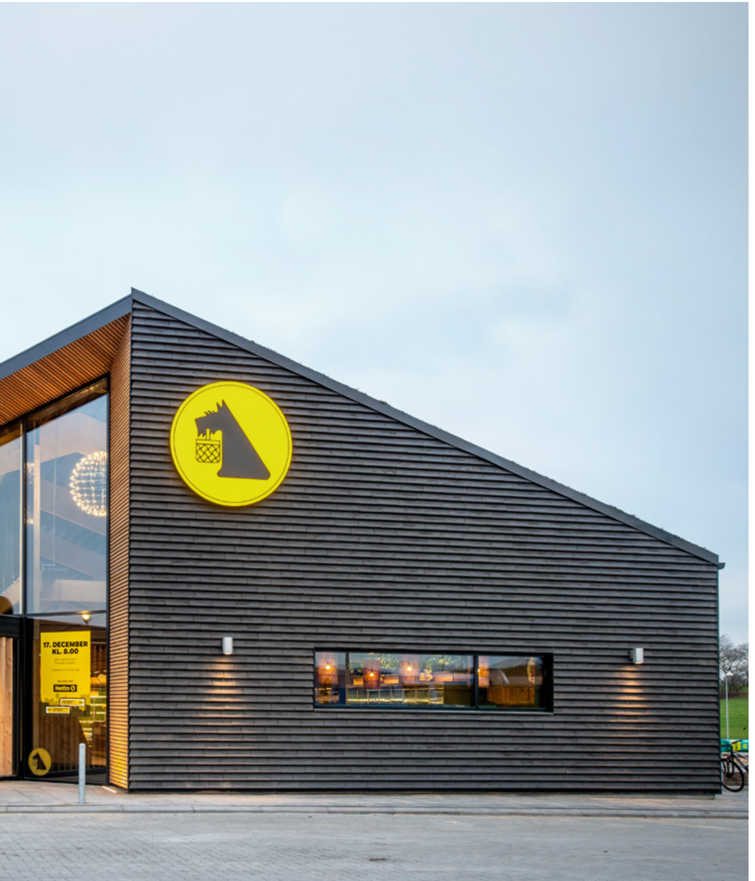
Netto supermarket, Horsens, Denmark C.F. Møller Architects Completion in 2020
